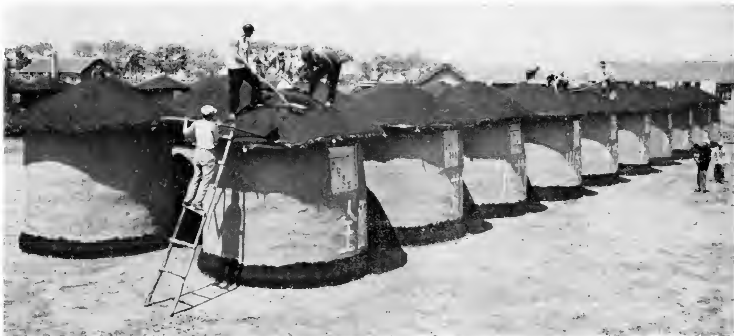
Shuangsheng brigade builds barns.
